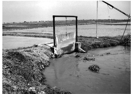
Contemporary culvert of irrigation system in Tien Hai district
