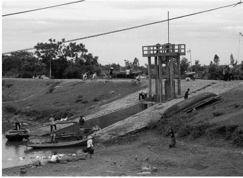
The main culvert takes water from the Tra Ly river to irrigation system
