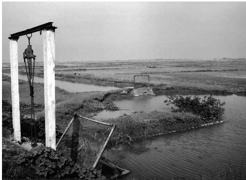
Smaller culvert take water to paddy field
